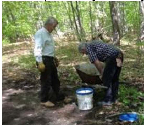
Carl Lombard and Joe Secondino on culvert repair.
