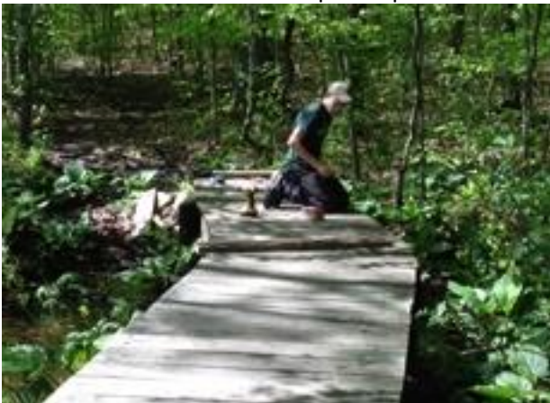
Chad on bridge repair.
